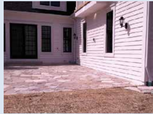
Patio with erosion control blanket
