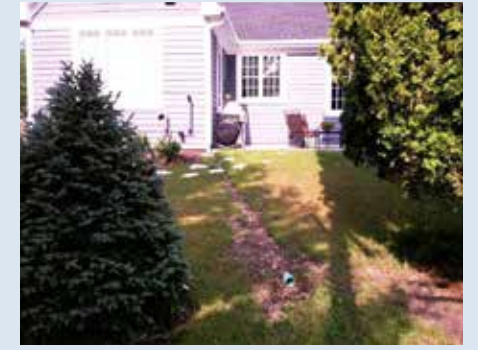
Downspout extension that creates a concentrated discharge near the property line
