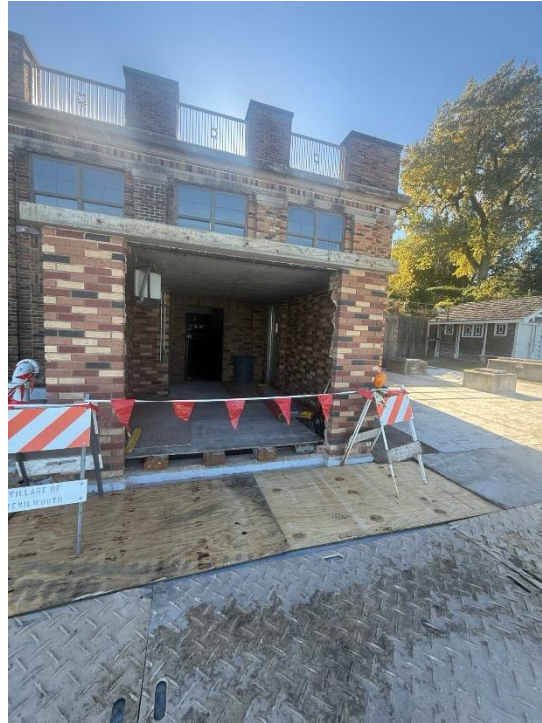
Figure 7: Brick removed from east side structure.
