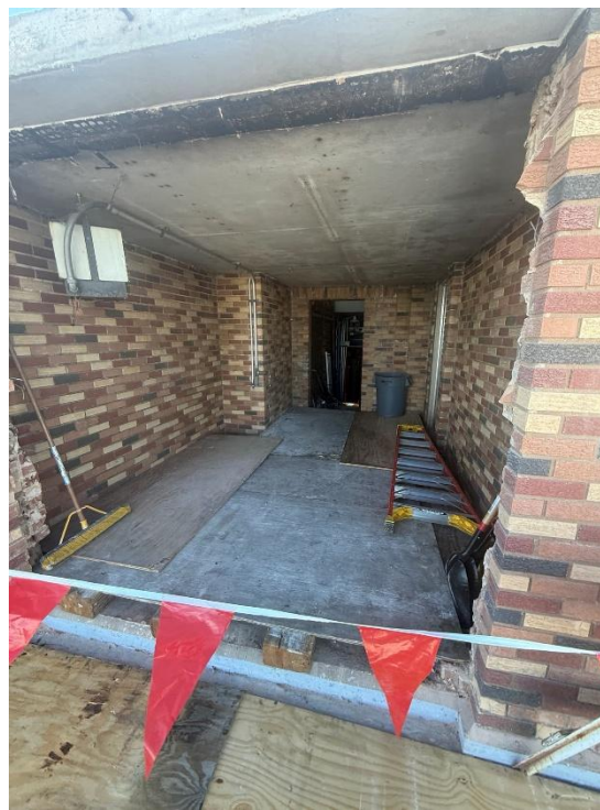
Figure 8: Additional view of east side structure.
