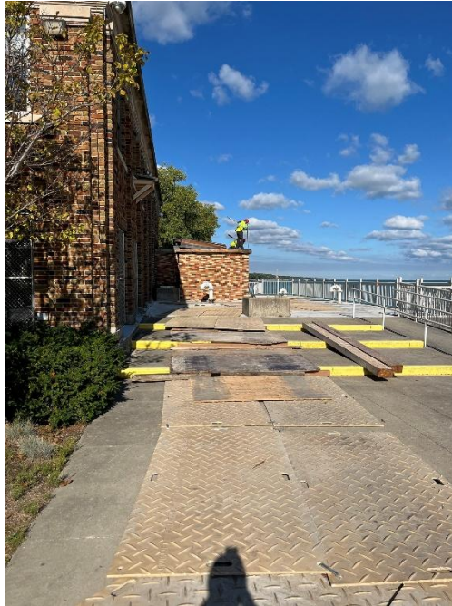
Figure 1: Protective plates placed to protect concrete that will remain.
