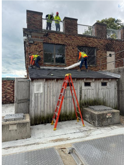
Figure 3: Removing roofing from connected wood structure.
