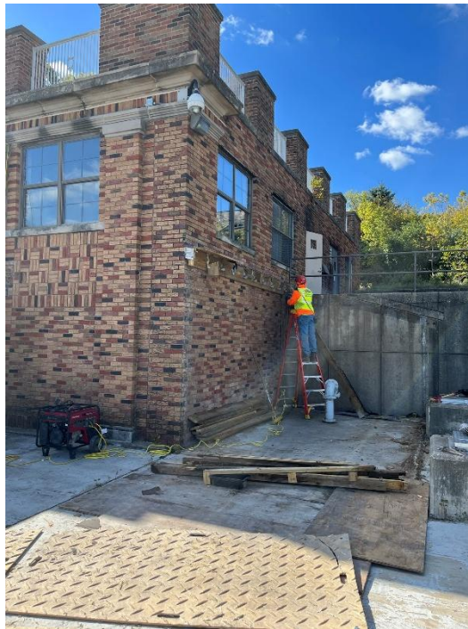
Figure 4: Wood structure being removed on north side of the building.
