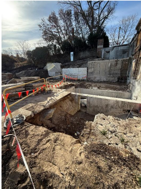
Figure 10: Additional view of the south side of the building.
