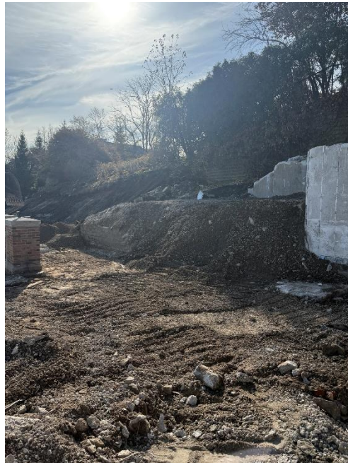
Figure 6: Grading being done on the bluff for new ramp design.
