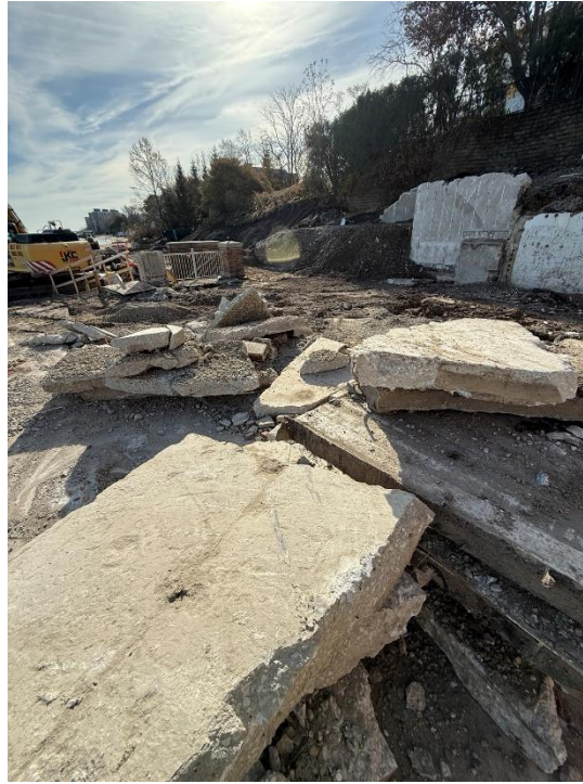
Figure 1: Concrete material to be removed.
