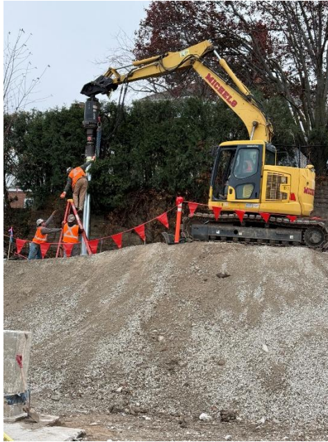
Figure 7: Second location of helical pier being installed for the new ramp.
