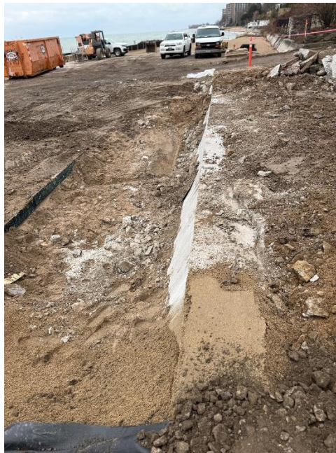
Figure 4: Excavated area on the south end of the site.
