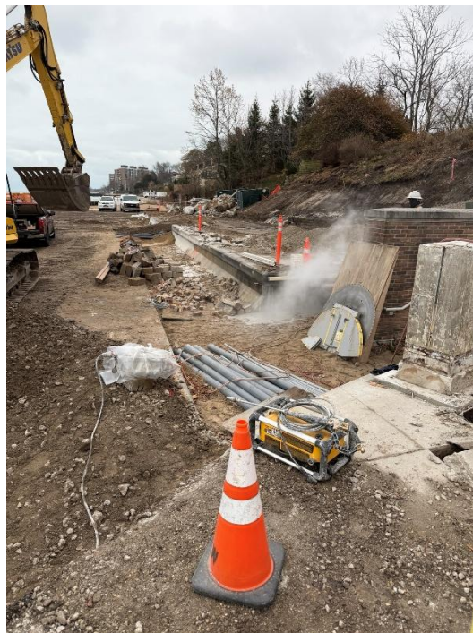
Figure 2: Removed concrete along the beach.
