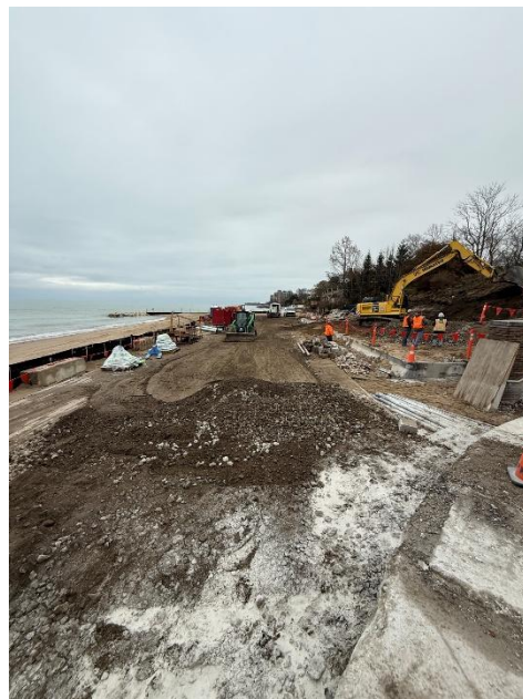
Figure 8: Last helical pier location being installed.
