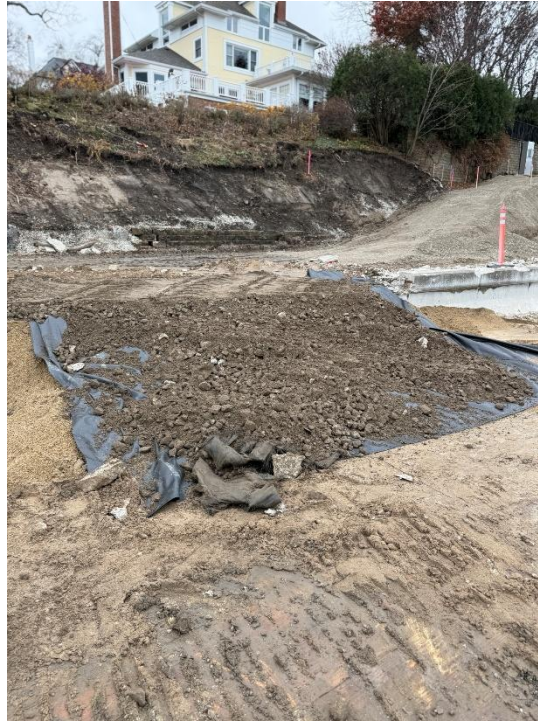
Figure 1: Excavated bluff being prepared for development.
