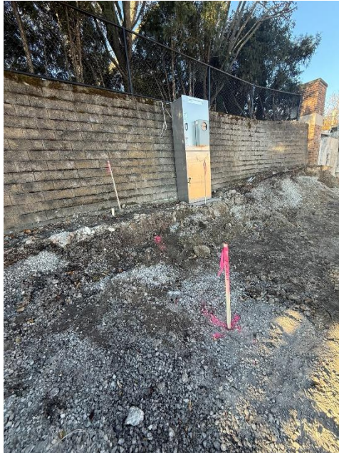
Figure 3: Stake marking the location for helical pier to be installed.
