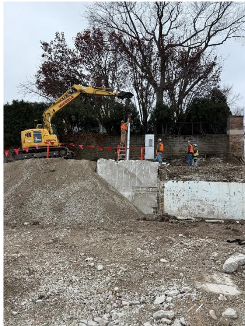
Figure 6: Equipment installing a helical pier.
