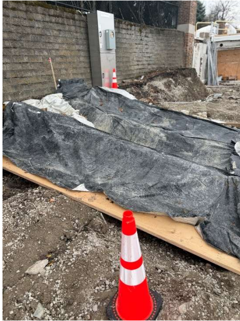
Figure 3: Protection of other excavated areas.
