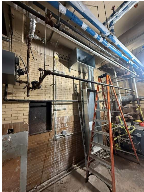
Figure 6: New cabinet installed inside the maintenance room.
