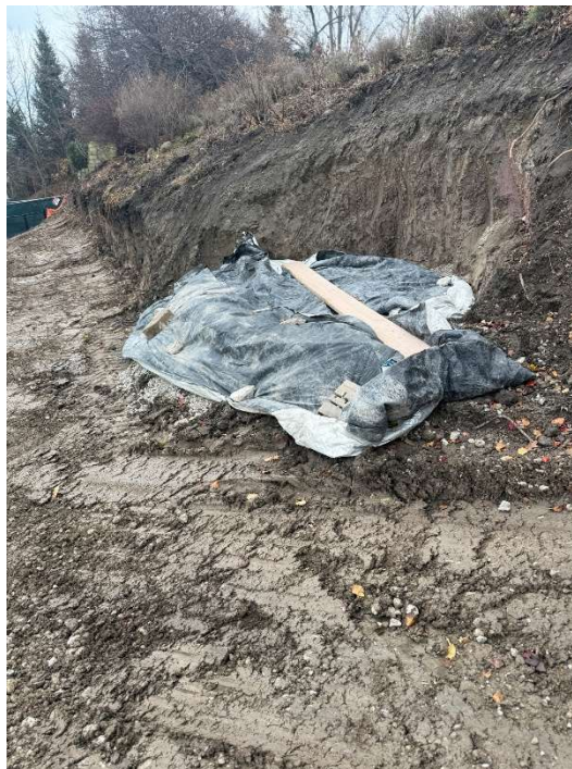
Figure 2: Protection over excavation in anticipating the cold and snowy weather.
