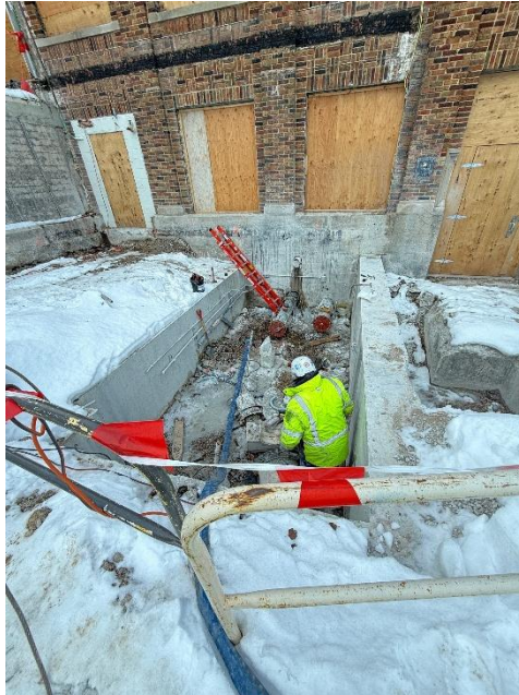
Figure 3: Removing existing piping under new foundation location.
