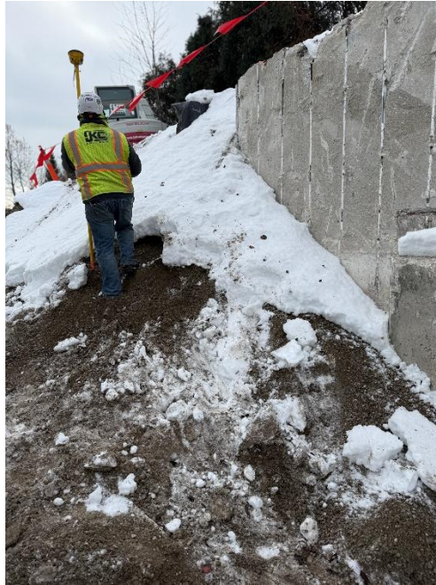
Figure 5: Excavators confirming grading of foundation wall.
