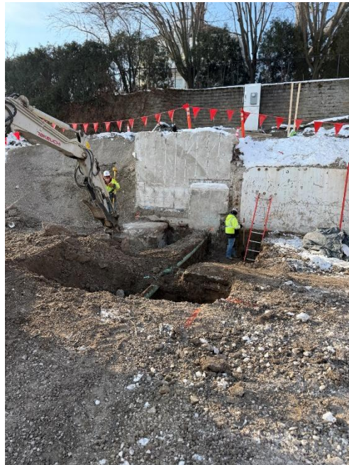
Figure 6: Excavations for new foundations.
