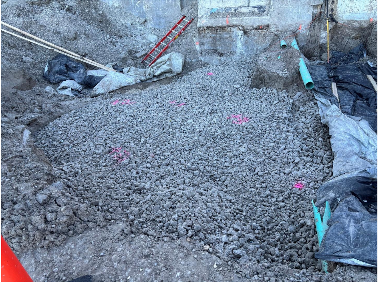
Figure 5: Filled in Silo to Grade
