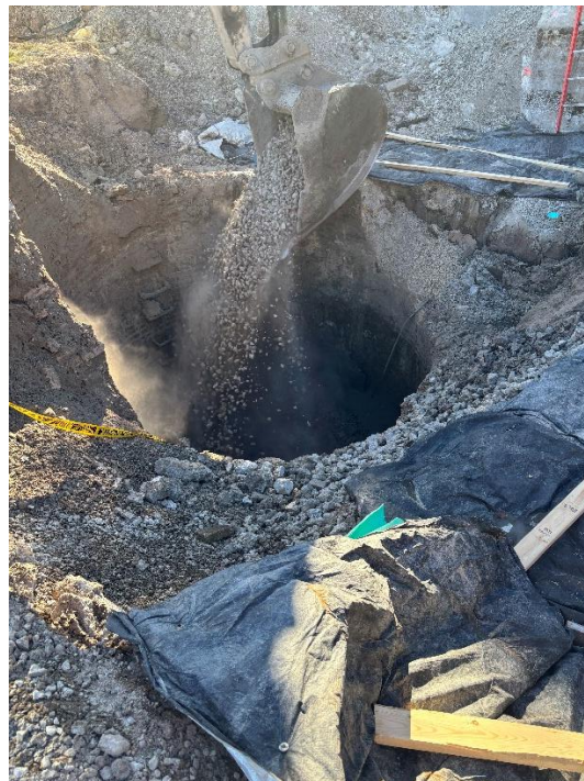
Figure 4: In progress Photo of Silo Infill
