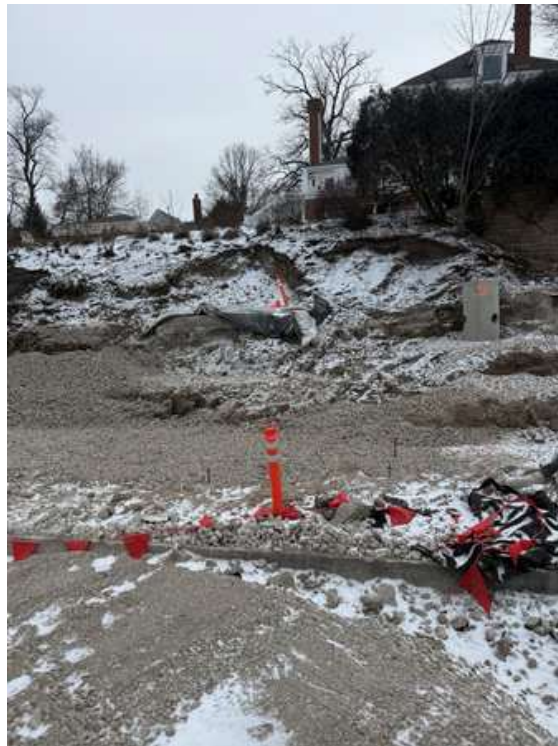
Figure 2: Rough Site Grading
