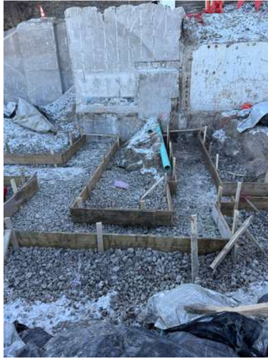
Figure 5: Additional Formwork and Site Utilities
