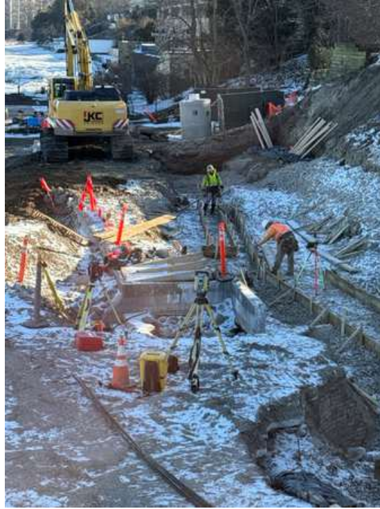
Figure 3: Ramp Formwork
