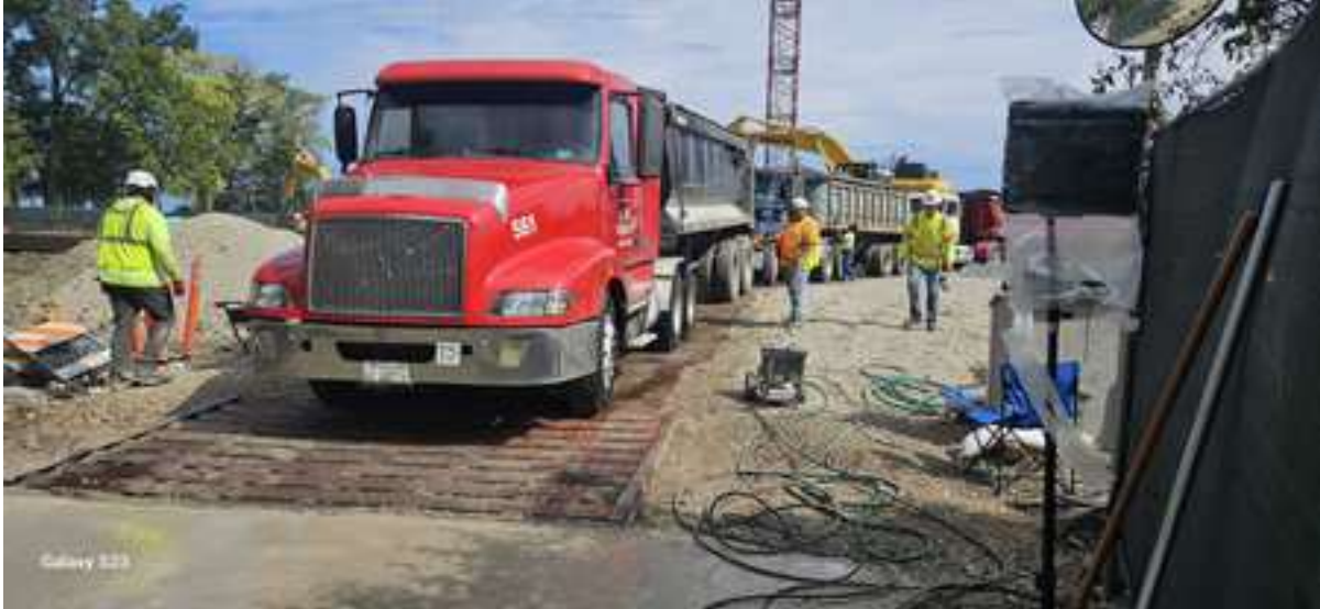
Figure 1: Installed Rumble Mats
