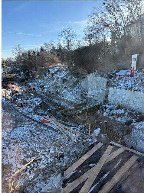
Figure 3: Framing for the foundations on the south end of the site.
