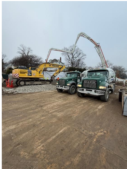
Figure 8: Pump trucks to pour concrete in difficult areas on the bluff.
