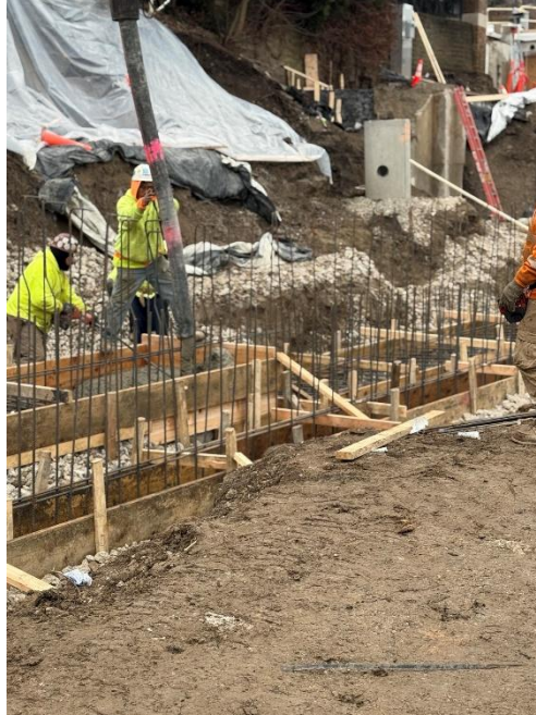
Figure 9: Pouring the concrete in the form foundations.
