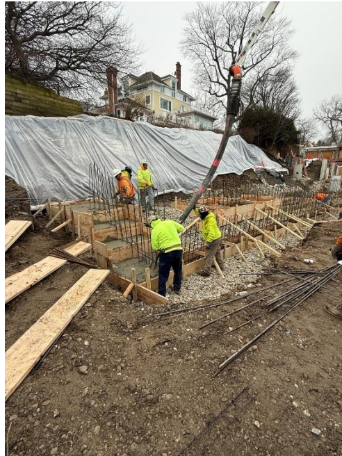
Figure 10: Additional view of concrete being poured.
