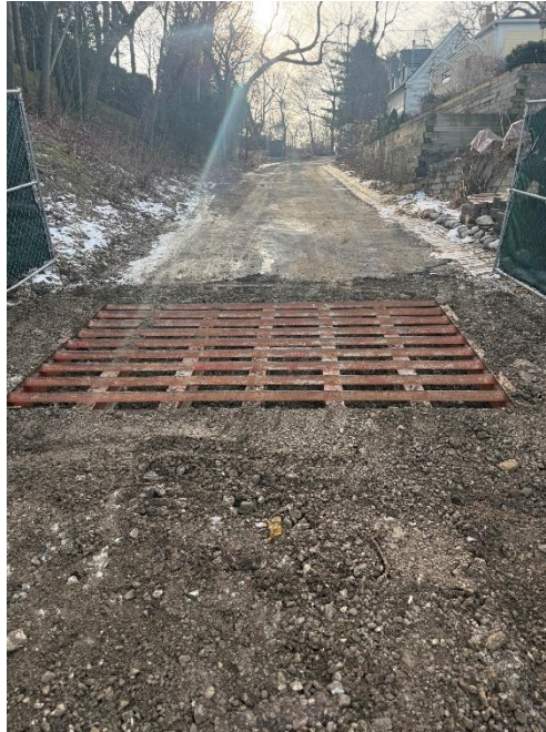
Figure 5: Matt installed on Devonshire to ensure clean streets.
