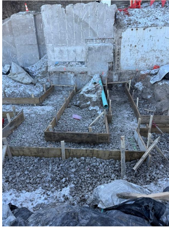
Figure 1: Framing for concrete foundation.
