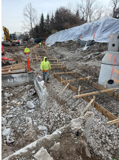
Figure 7: Additional view of rebar in concrete forms.
