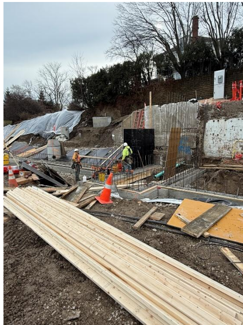
Figure 12: Preparing forms for the concrete foundation walls.
