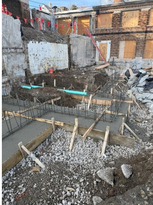
Figure 11: Concrete foundations poured.
