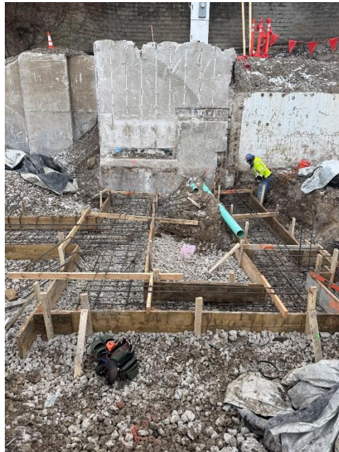
Figure 6: Rebar installed in framing.
