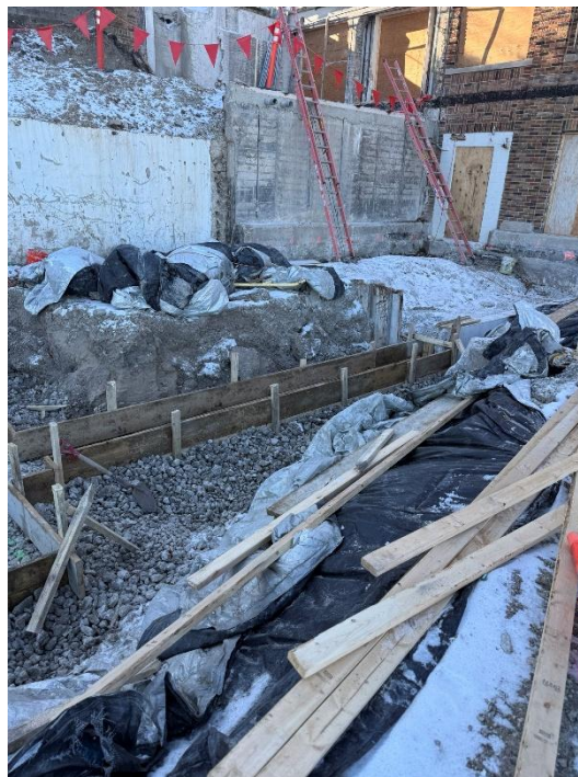
Figure 2: Additional view of the foundation framing.
