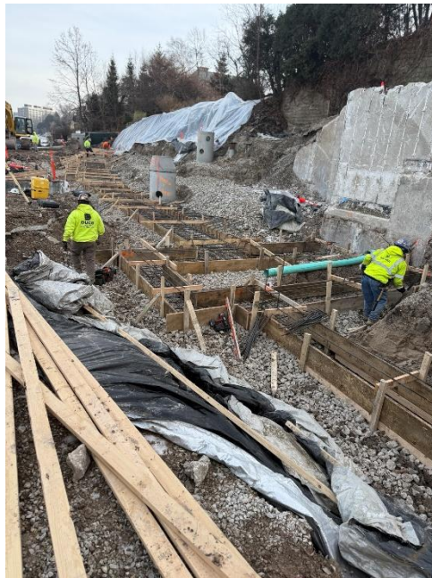
Figure 4: Framing and foundations being installed in preparation for concrete pour.
