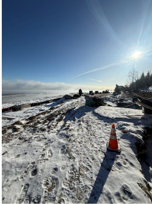
Figure 1: View of site conditions in sub-zero temperatures.
