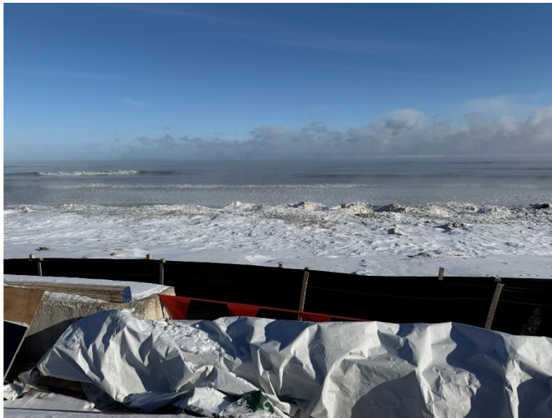
Figure 2: View of the site conditions facing the Lake.
