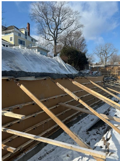
Figure 4: Framing for concrete walls.
