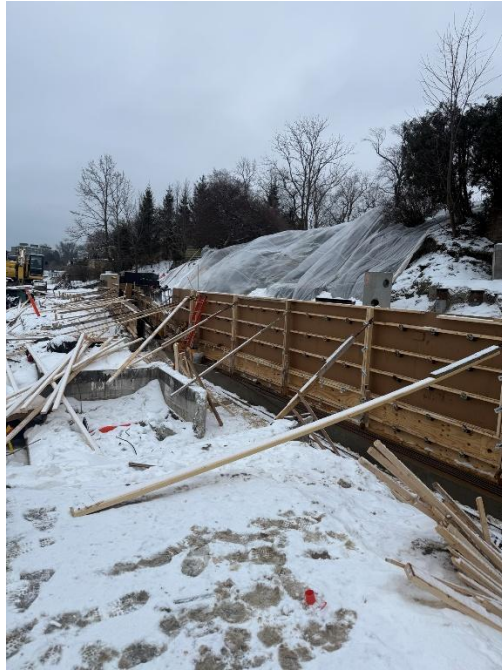
Figure 3: View of concrete forms on the south side of the site.
