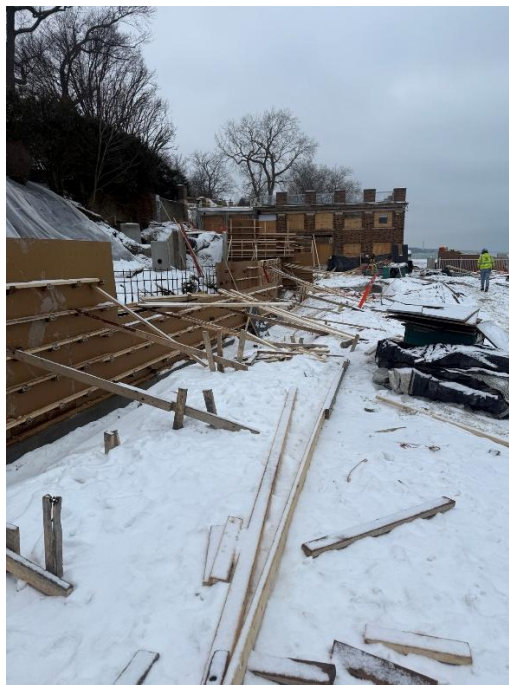
Figure 2: Snow being removed from inside the concrete forms.
