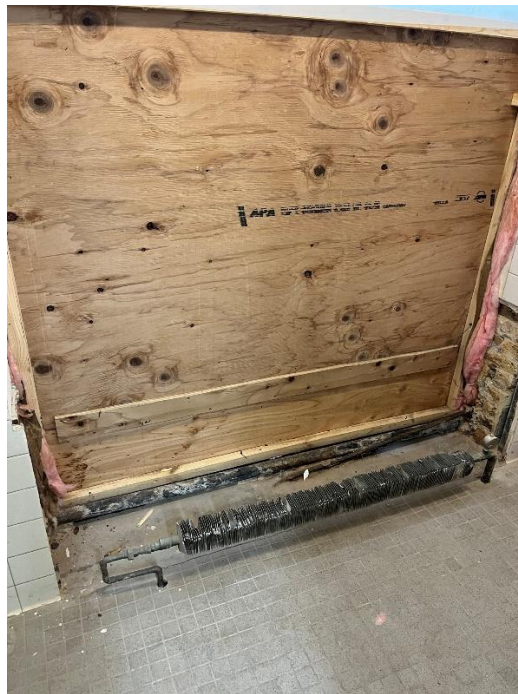
Figure 4: Window and brick removed to allow for measuring of new entrance.
