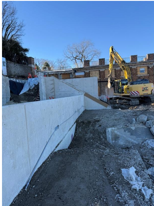
Figure 5: New concrete facing North.
