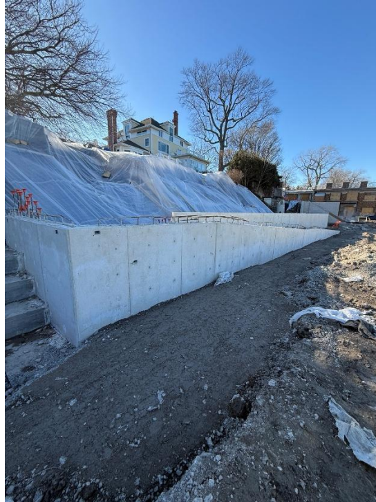
Figure 7: Concrete on the south side of the site.
