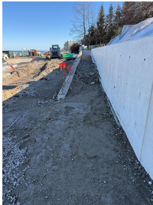
Figure 4: View of concrete ramp walls.
