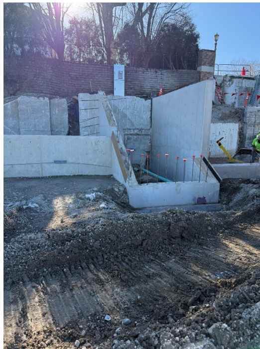
Figure 2: Additional view of new concrete poured for the ramp.
