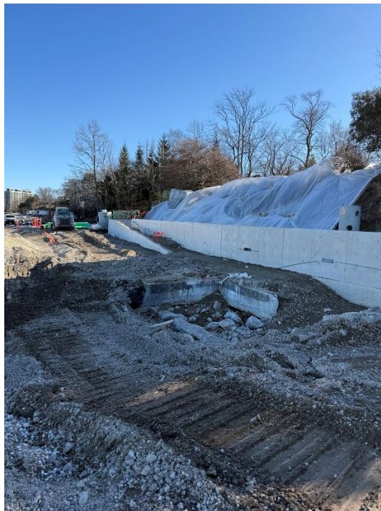
Figure 6: View of ramp concrete on the south side of the site.
