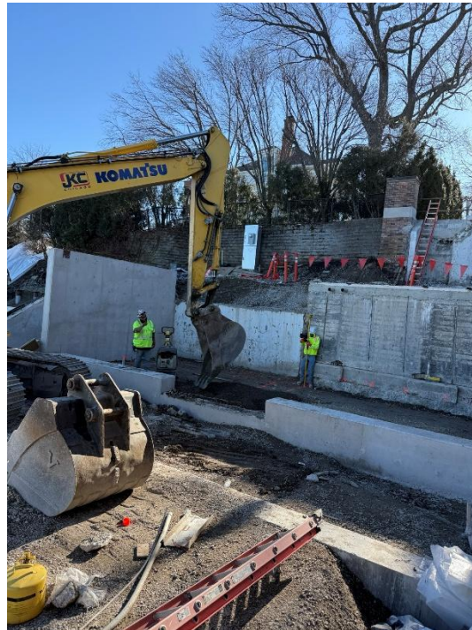
Figure 3: Backfill occurring behind new concrete.
