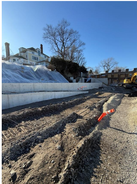
Figure 8: Addition view of ramp concrete.
