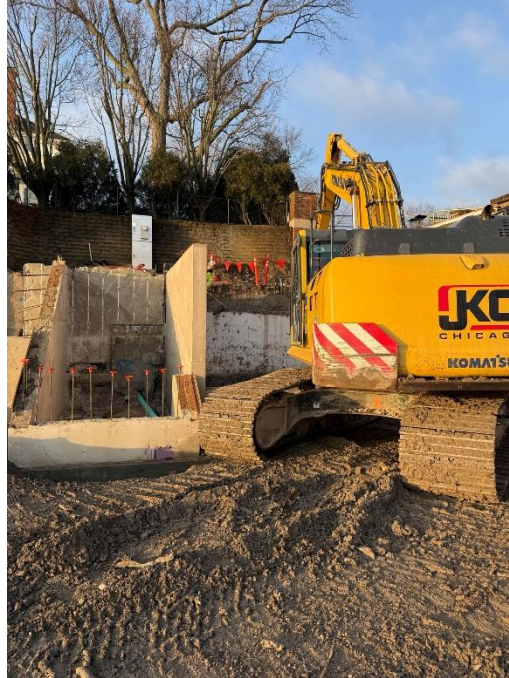
Figure 1: Concrete walls for new stair well.
