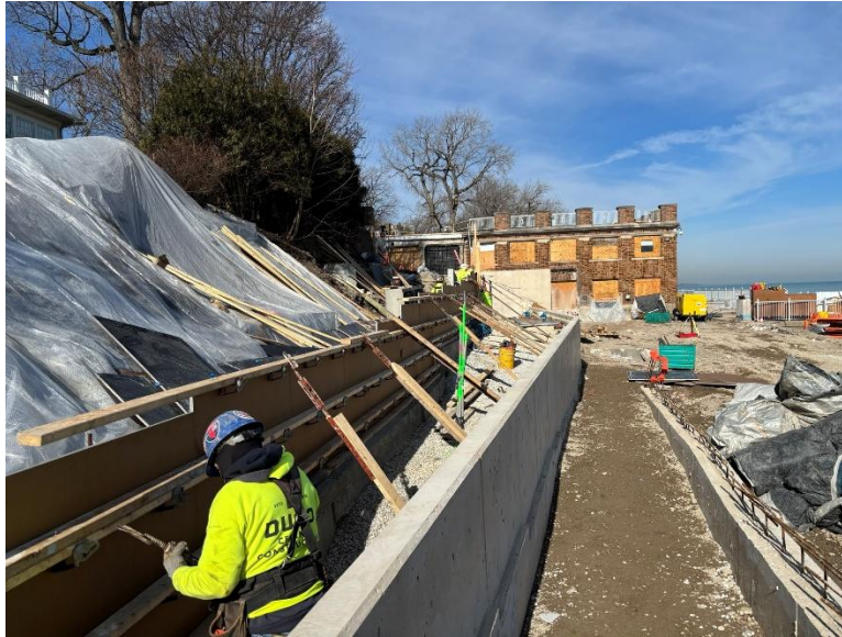
Figure 3: Additional framing being installed for the next concrete pour.
