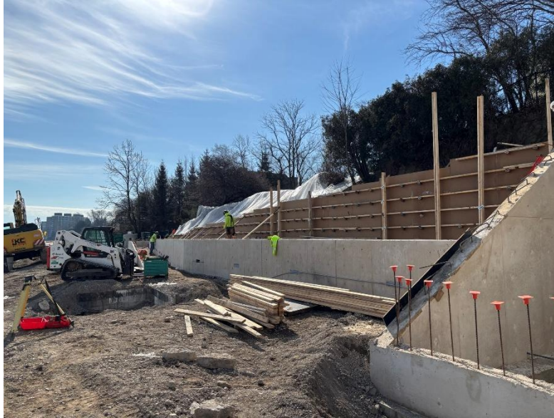
Figure 1: Concrete framing for additional ramp walkway.
