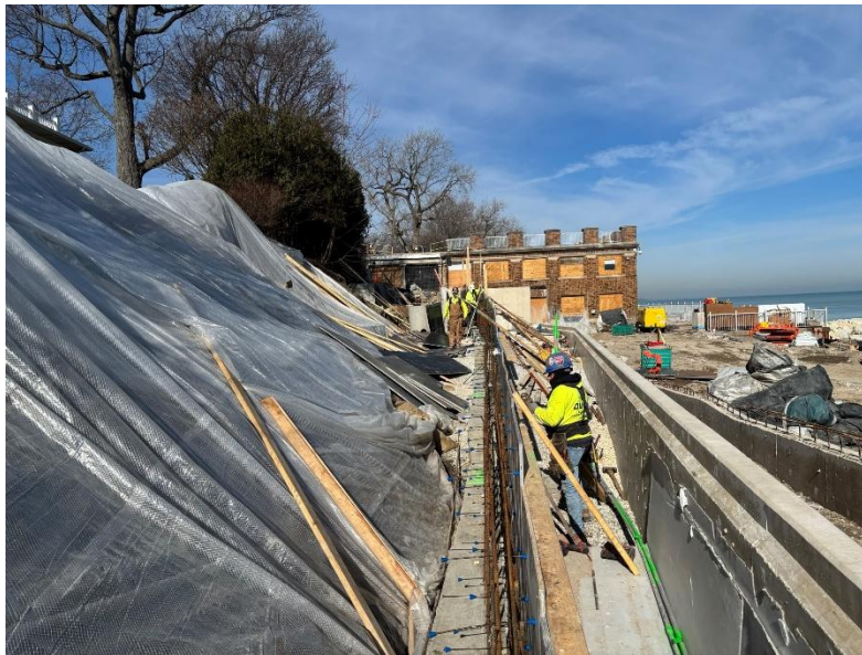
Figure 4: View of concrete ramp walls.
