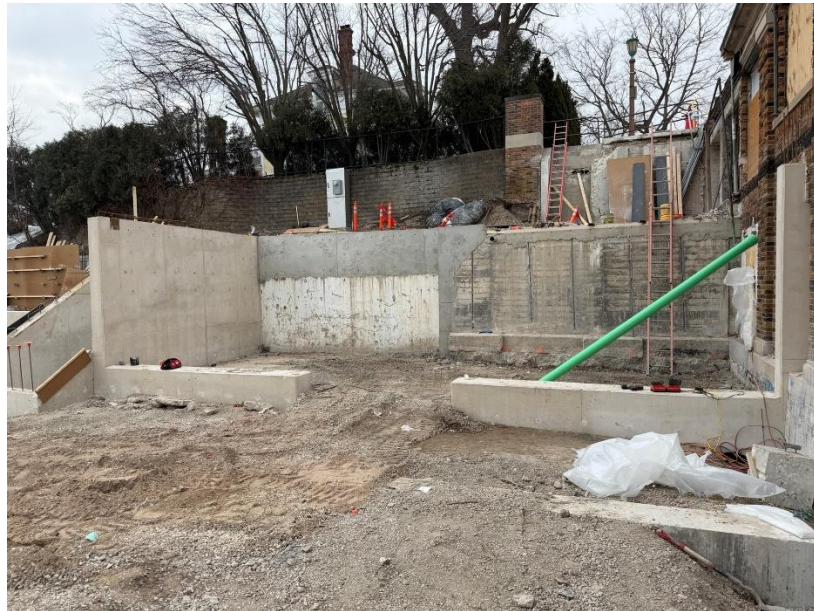
Figure 6: Concrete outline of new bathroom building.
