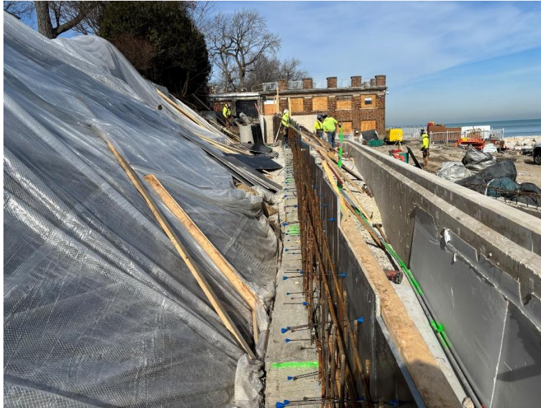
Figure 2: Rebar and framing installed for the next concrete pour.
