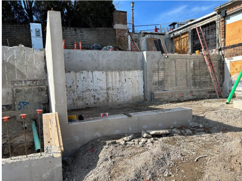
Figure 5: New rebar installed on the building.
