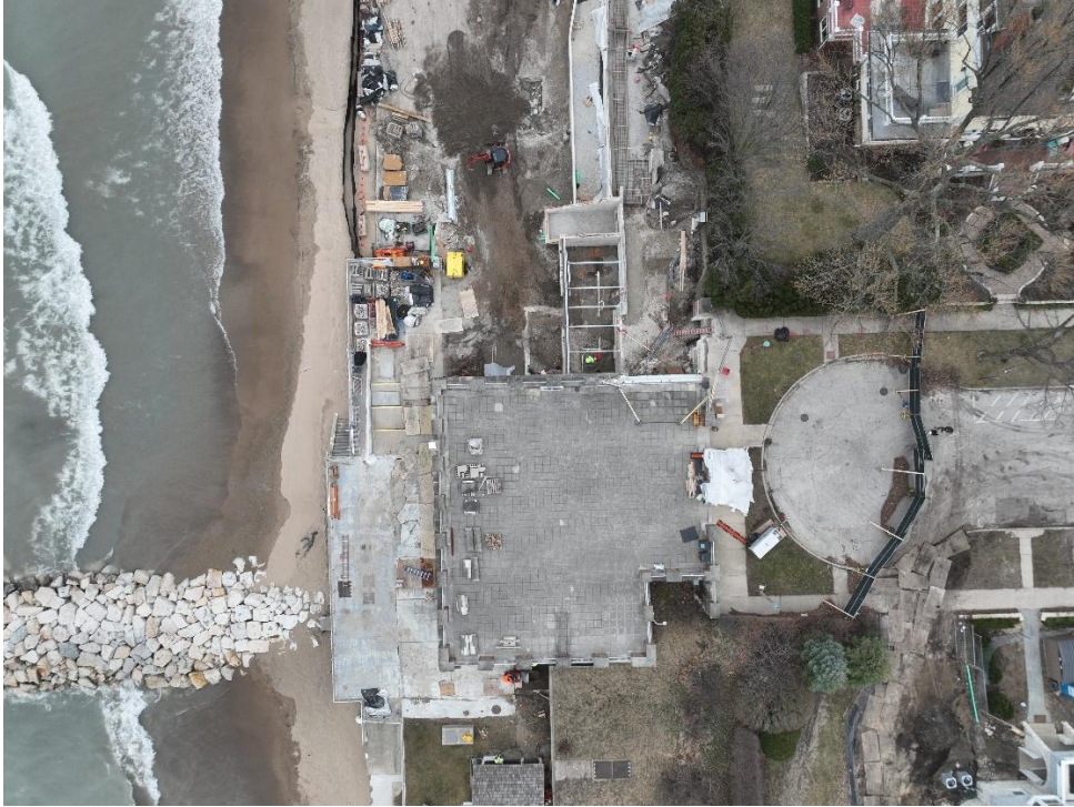
Figure 7: Overhead site photos.
