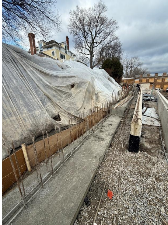
Figure 5: Framing for more concrete that will be poured.
