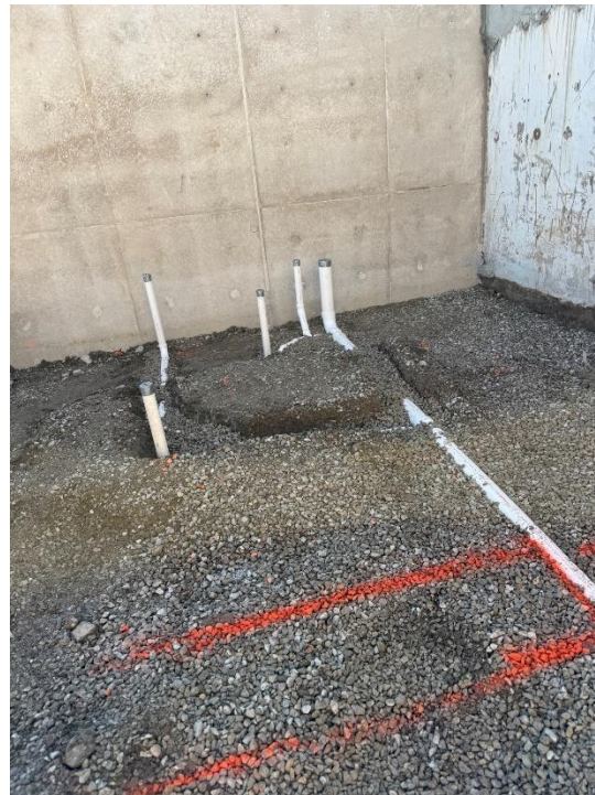
Figure 4: Install underground plumbing in the new Bathhouse.
