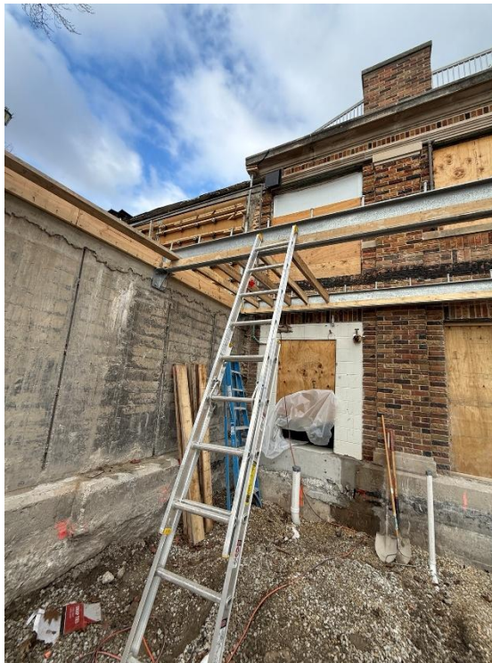
Figure 6: Preparing the roof of the Bathhouse.
