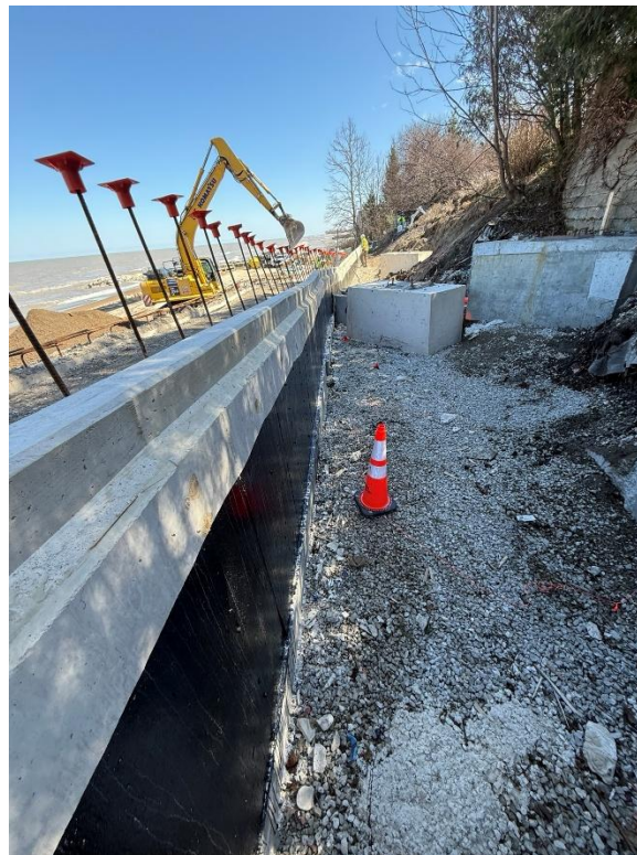
Figure 6: Ramp wall and foundations.
