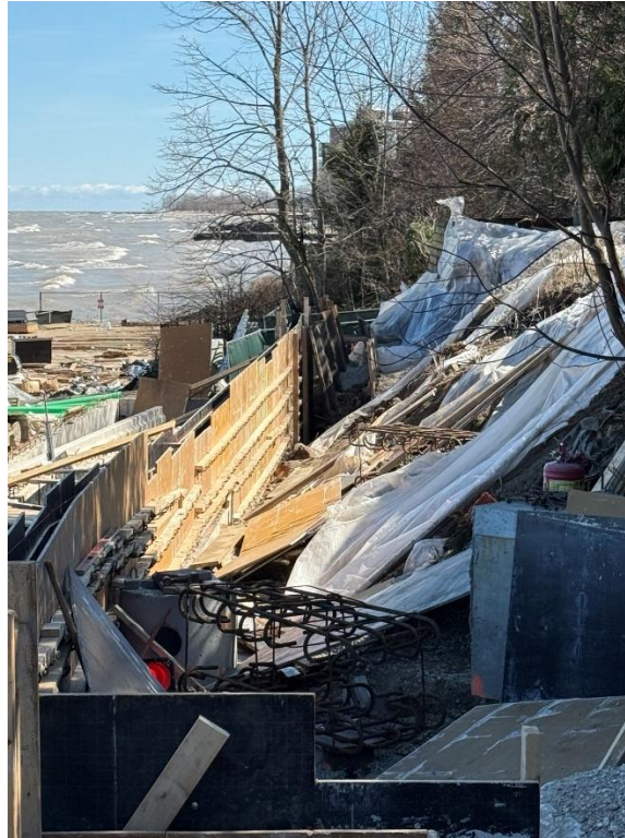
Figure 5: Additional framing for concrete.
